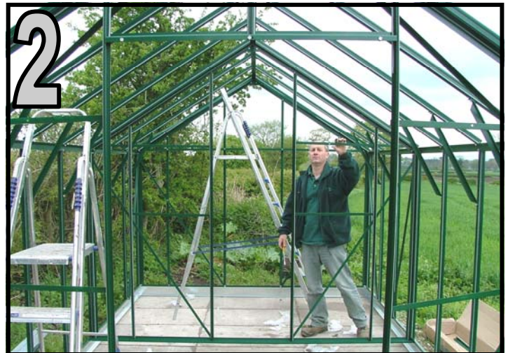
2 Add vertical glazing bars and bracings.
