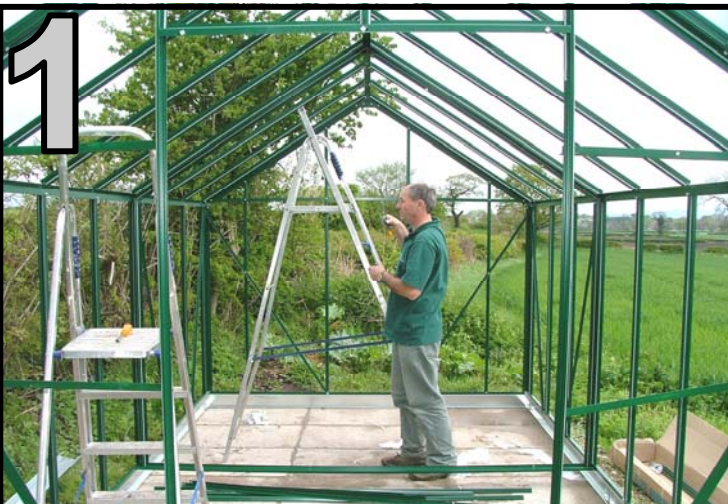
1 Join Base cill to the special partition side / roof sections.
