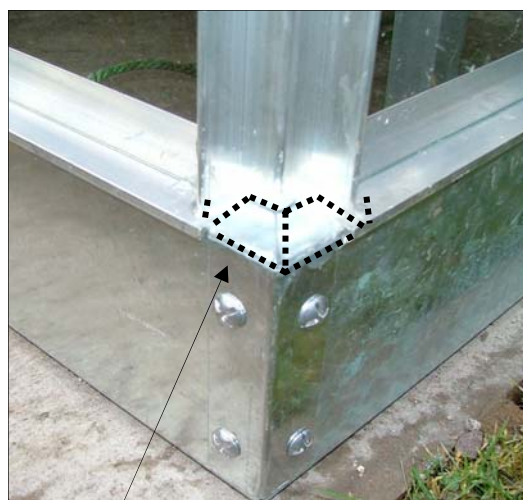
Silicone around base corners and mid-joints (if applicable).
