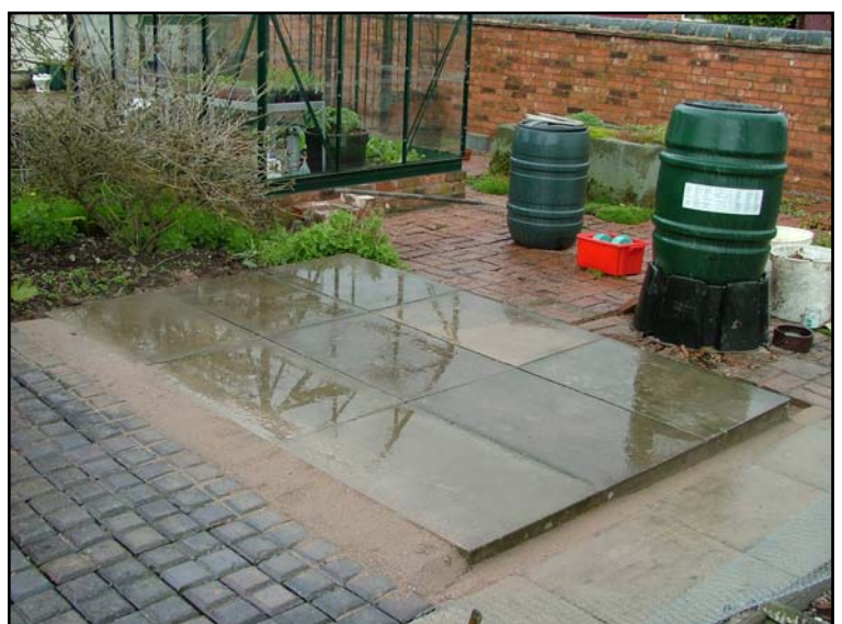
A 6x8 slab base: ideal for a 5x6 greenhouse. Remember that your greenhouse is a few inches bigger than the nominal
